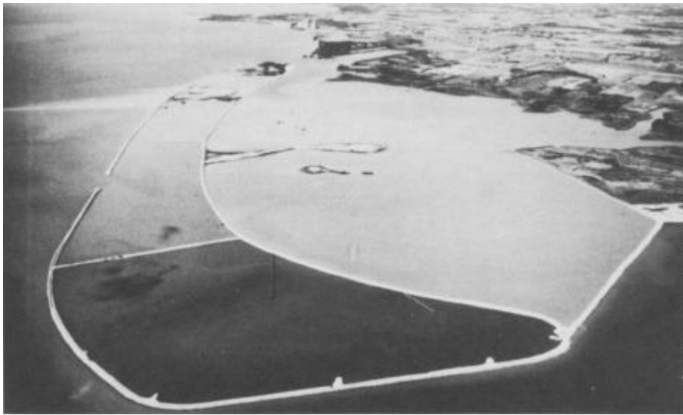
Figure 14-2. Pointe Mouillee, in western Lake Erie, is a CDF for contaminated dredged material that also serves as a multipurpose beneficial use site
